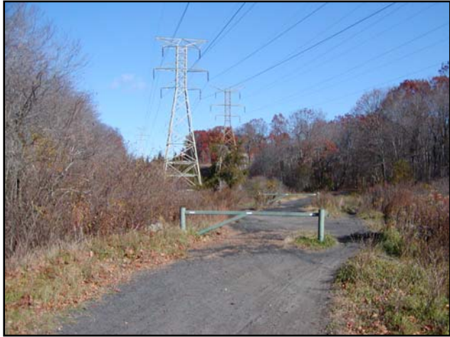
Larkin State Trail at power line crossing
